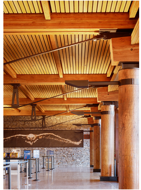
Douglas-fir columns, premium-appearance glulam beams, a tongue-and-groove ash wood ceiling, and natural stone wall give visitors a warm Wyoming welcome.
